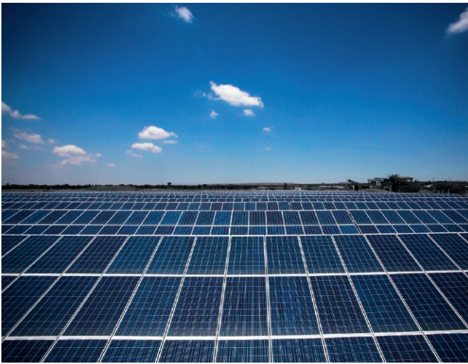
Fig. 2. Zimbi project in South Africa.
